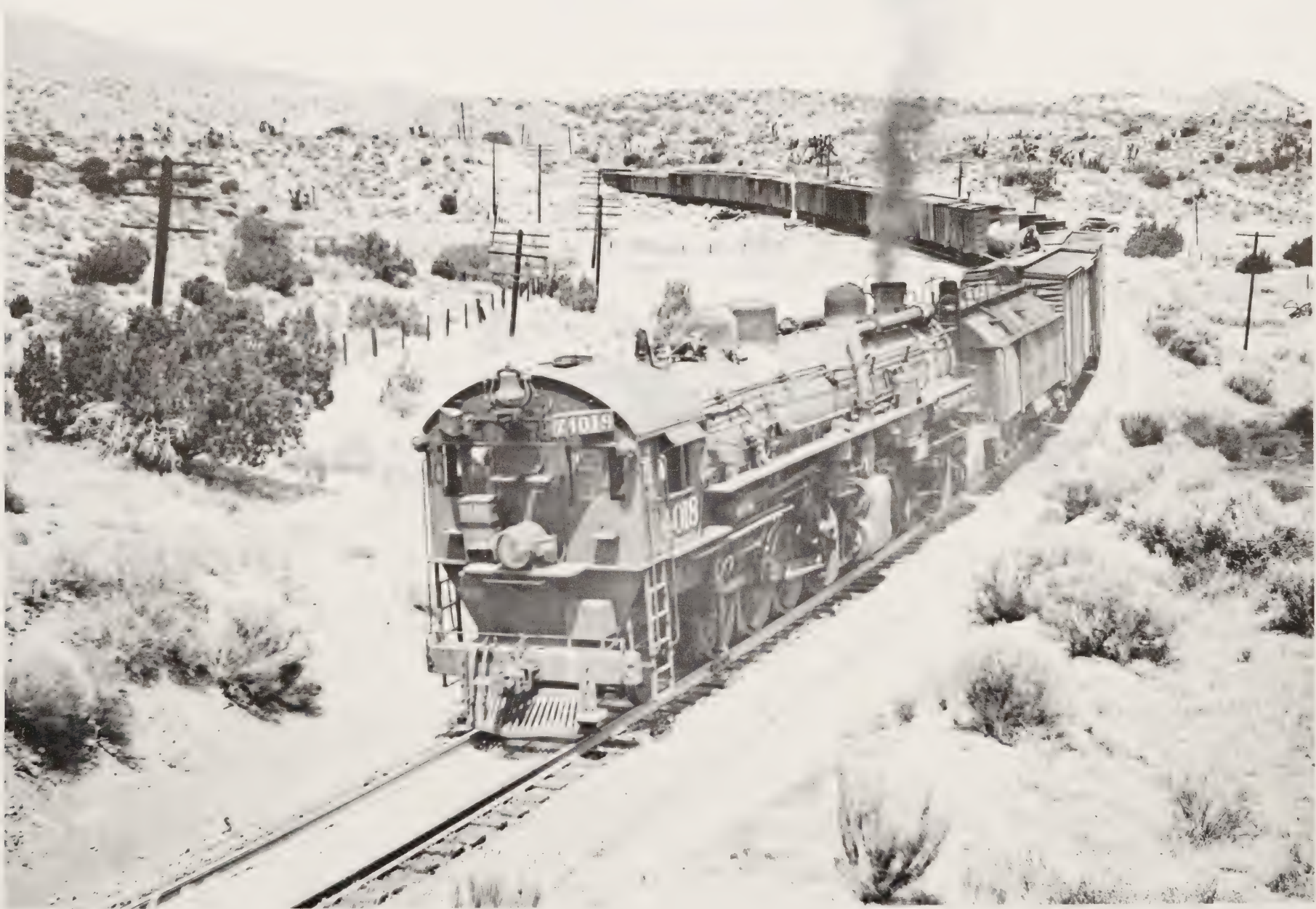
Mallet Locomotive of the 2-8-8-2 Type Moves Beyond Antelope Valley With a Los Angeles Bound Manifest.
